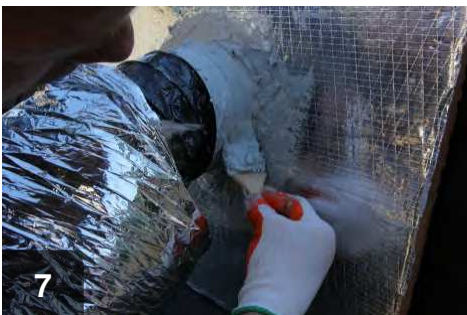
7 Coat seam with mastic
