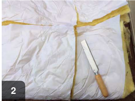
2 Wrap blanket around tank and mark it where it overlaps. Add two or three inches and cut off using a straightedge and raz
