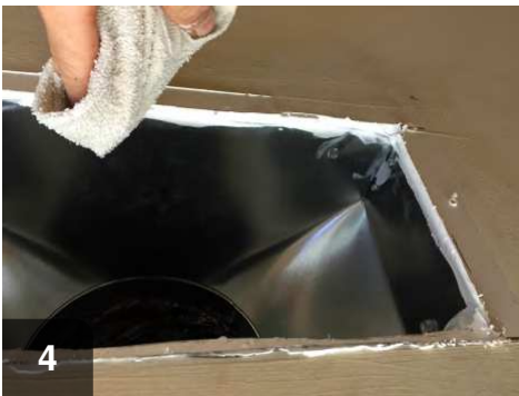
Wipe away excess caulk (use water on siliconized acrylic, alcohol on silicone, and solvent on polyurethane caulk)
