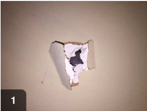
1 Replace any missing insulation and repair holes in vapor barrier
