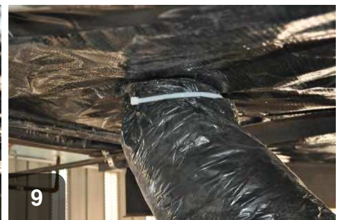
9 Use band tensioner to ensure that insulation and casing remain tight against belly
