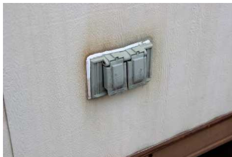
Exterior electrical outlet sealing.
