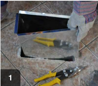
1 Replace damaged ducting if necessary
