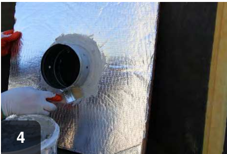
4 Coat joint between starting collar and duct board with mastic. Liberally coat the metal collar where flex attaches
