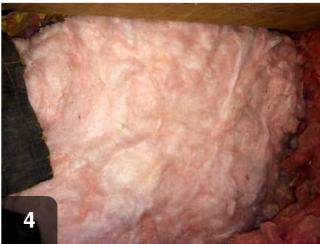
4 Replace or reinstall fiberglass belly insulation
