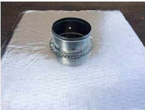
Insert the starting collar, bend tabs over and install at least 3 screws through the collar, duct board, and backer ring
