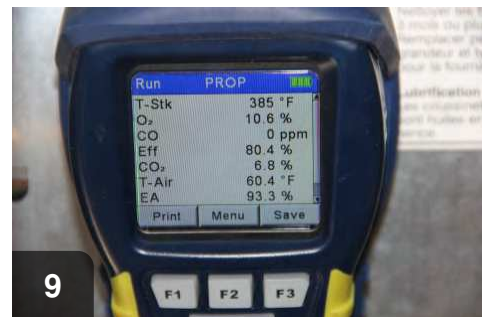
9 Measure flue gases at steady state and record readings. Turn off the unit being tested per manufacturers instructions.
