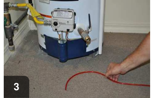
3 Place test hose by combustion appliance
