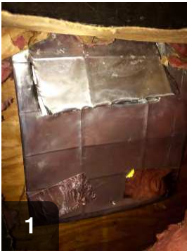
1 Thoroughly clean duct with solvent before applying foil tape and mastic
