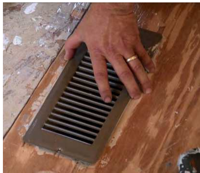
Install a new grille on the rebuilt boot.
