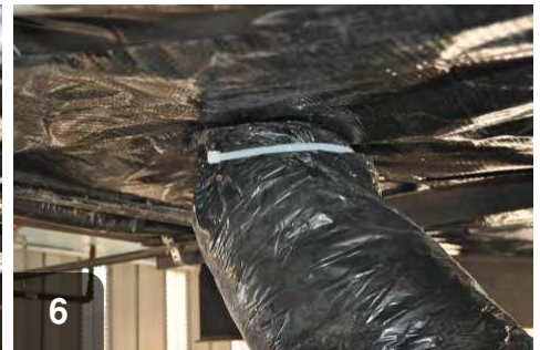
6 Secure insulation and casing in place using tie band and band tensioner
