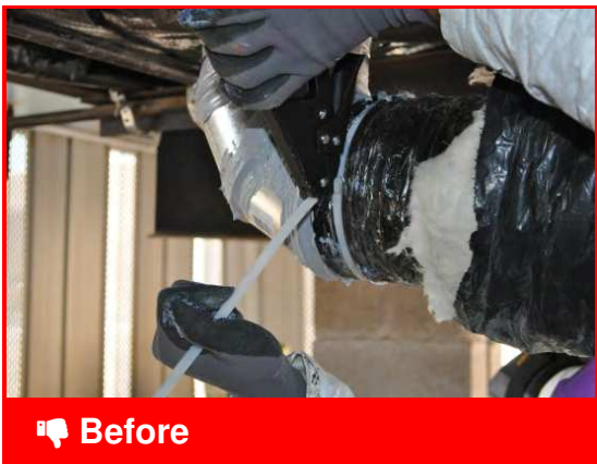
This elbow has been sealed, but is not insulated.
