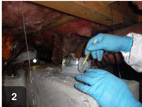
2 Apply mastic to metal collar
