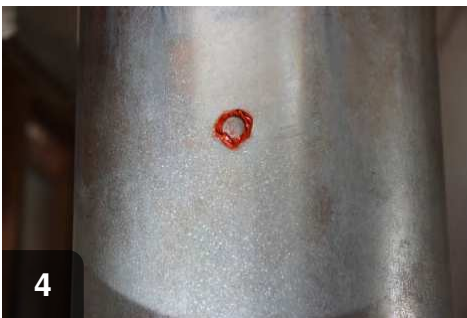
Apply high temperature sealant to the perimeter of the plug.
