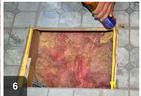
6 Apply sealant to mounting surfaces
