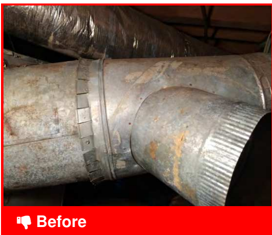
Unsealed metal ductwork
