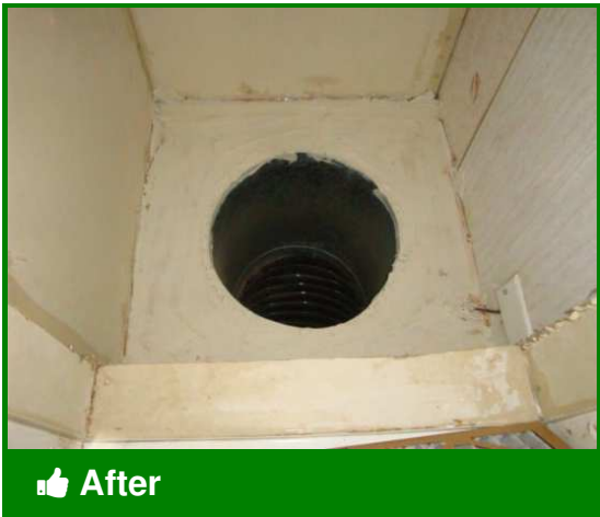
Closet prepared for furnace installation
