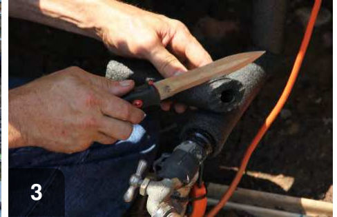
3 Measure and cut insulation to fit water lines. Miter insulation at elbows and tees
