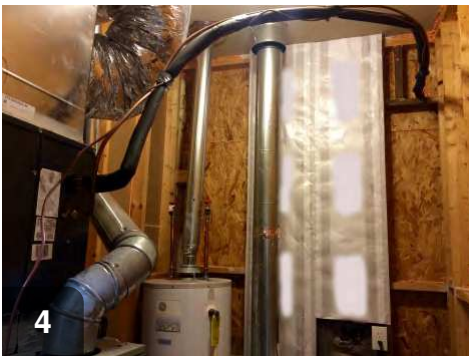
4 Complete installation by adding supports and fasteners as required for stability and durability
