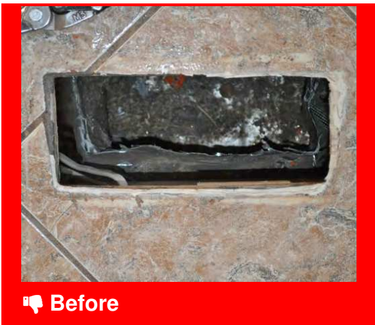
Unattached ducts are useless
