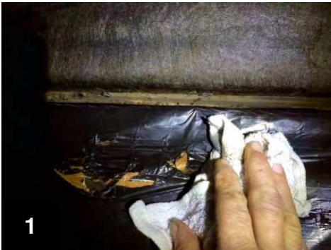
1 Clean belly wrap before air sealing
