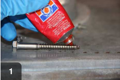
Apply high temperature sealant to the bolt, so that both holes will be sealed.
