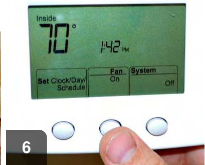
6 Is the air handler on?
