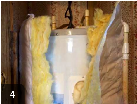
4 Pull insulation blanket around the tank
