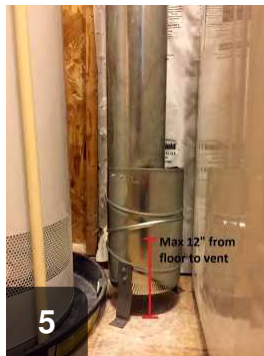
5 Terminate the low vent within 12" of the floor. This one is mounted inside a section of larger diameter metal duct
