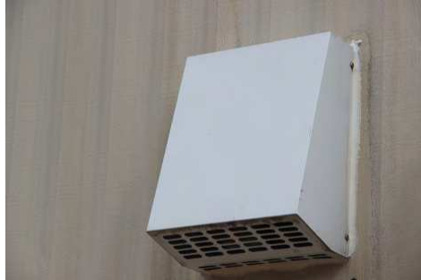
Through the wall exhaust fan sealing.
