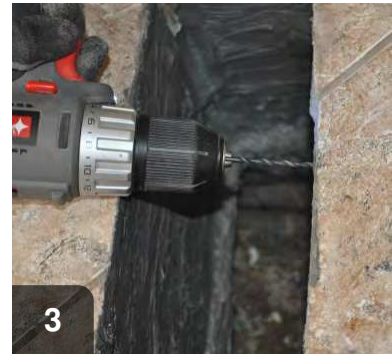
3 Drill pilot holes for metal fasteners
