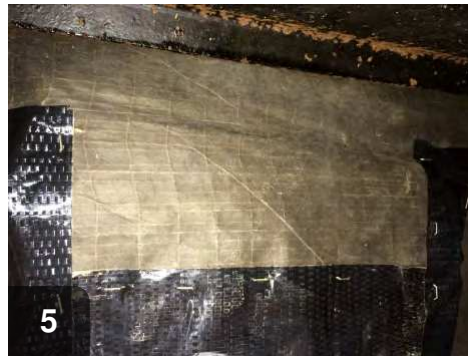
5 Apply belly repair tape and fasten with outward clinching (stitch) staples. Spray adhesive will help adhere the tape
