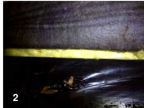
2 Stuff wide gaps in the marriage line with fiberglass insulation or foam backer rod before applying sealant
