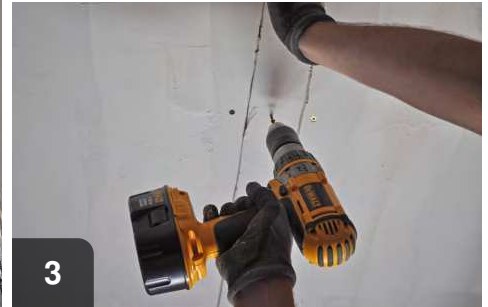
3 Cut drywall and fasten in place
