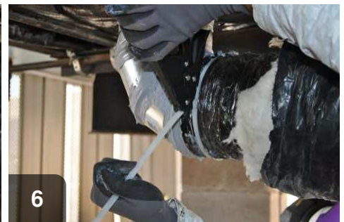
6 Fasten inner inner with tie band using band tensioner
