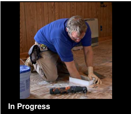
Here the worker is rebuilding a hard connection to the trunk line.
