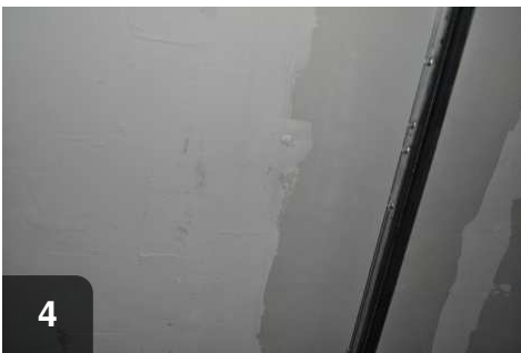
4 Add joint tape and first coat of joint compound
