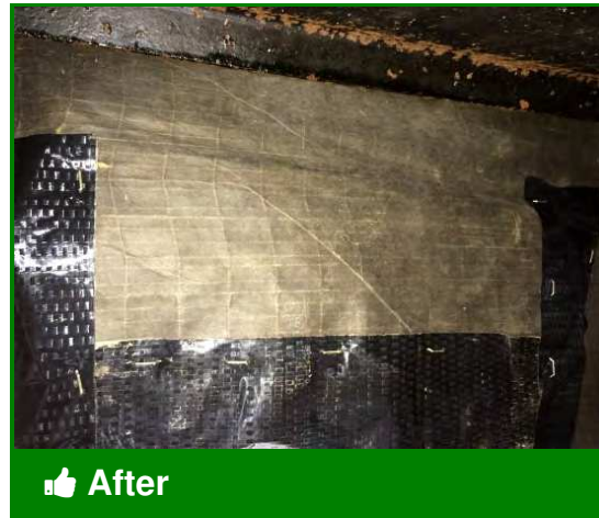
Repaired, insulated, and sealed access hole in manufactured home duct and belly
