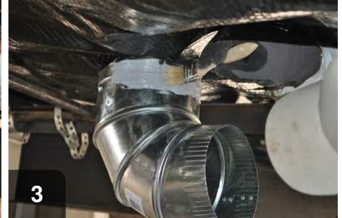
3 Apply mastic at metal-to-metal connection
