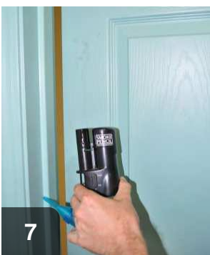
7 Check interior doors for pressure differential either using smoke pencil or hand
