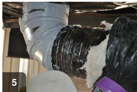
5 Slide inner liner onto flange with sealant
