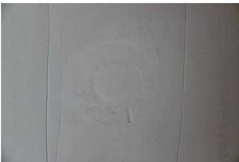
Backing or infill substrate may be needed for some wall patches.
