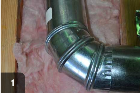
1 Prepare work area by assessing any safety concerns and cleaning duct surface
