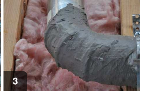
3 Apply UL 181 mastic to seal joint
