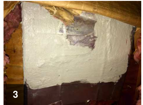
3 Overlap foil tape with mastic by at least one inch on all sides
