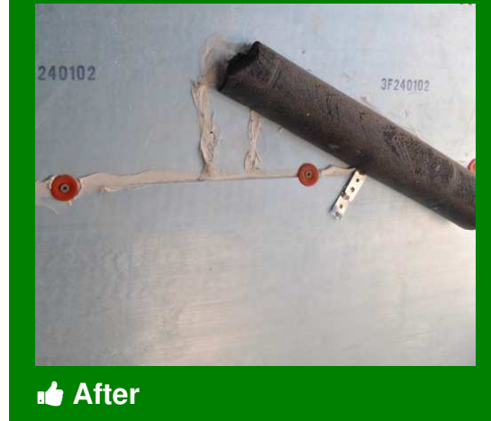
In addition to fiberglass batt insulation, a rigid air barrier will be sealed and mechanically fastened in place
