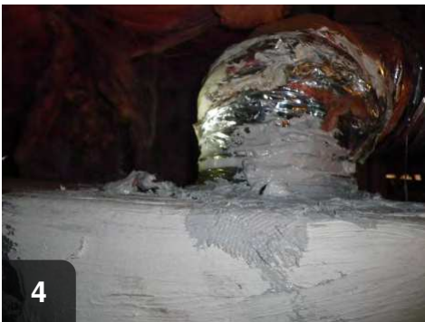
4 Apply additional mastic over zip tie and edge of flex duct liner
