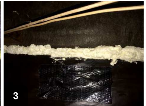
3 Apply foam or caulking over backer
