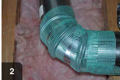
2 Wrap joint with fiberglass mesh tape
