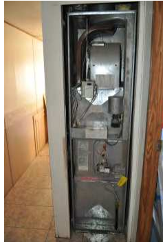
Test undiluted flue gases in induced-draft furnaces
