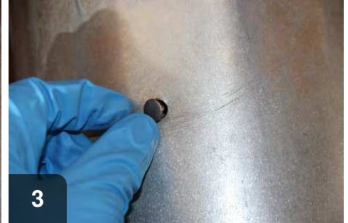
If sealing each wall individually, insert the plug into each hole.
