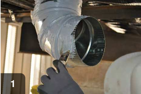
1 Apply mastic to flange
