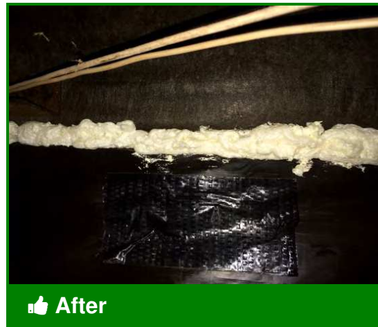
Completed air sealing at marriage line
