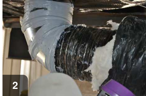
2 Slide inner liner onto flange with sealant
