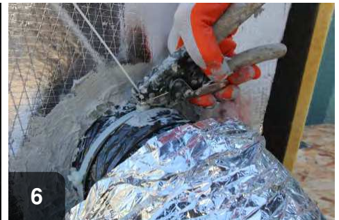
6 Secure with properly tensioned zip tie.
