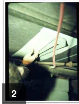
Seal around penetrations with compatible materials like foam board, belly board, house wrap, or Flex Mend (tm)
