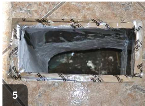
5 After securely fastened, duct should be sealed with mesh and mastic
