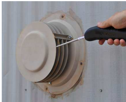
Test accessible exhaust outlets for direct-vent appliances
