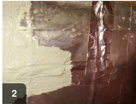
2 Secure edges of repair with foil tape and then liberally coat with mastic
