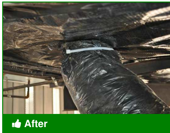
Fitting has been sealed and properly insulated.
