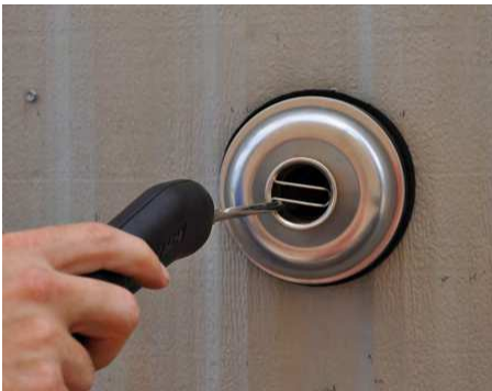
Test accessible exhaust outlets for power-vented appliances
