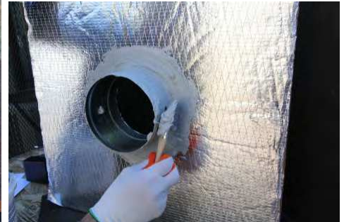
Apply mastic liberally and install flex duct
