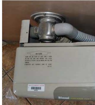
Ensure new combustion appliances are vented properly
