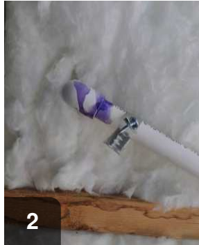
2 Notch insulation around pipes, blocks, and other obstructions
