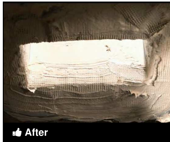
The duct has been sealed, ensuring proper airflow to the home.
