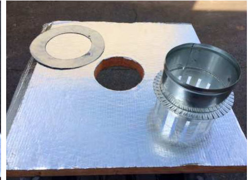
Select starting collar with tabs matching the thickness of the duct board
