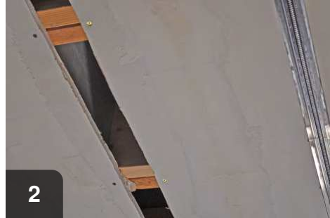
2 Prepare the hole by cutting the edges clean and square
