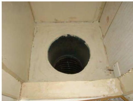
Apply mastic to inside seams of plenum
