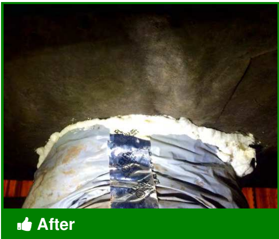
Crossover duct with vapor barrier mended and sealed to manufactured home belly
